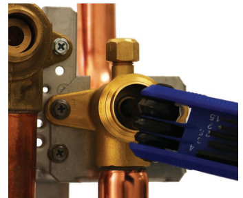
Figure 50: Opening the Service Ports.
