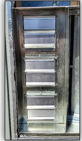
Figure 10: Rotate three (3) barometric relief dampers.
