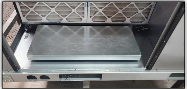
Figure 9: Insert the economizer (Step 4).
