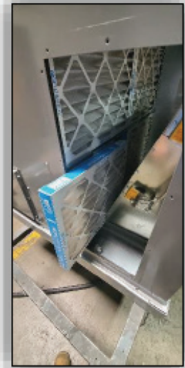
Figure 22: Pulling Out the Bottom Filter.
