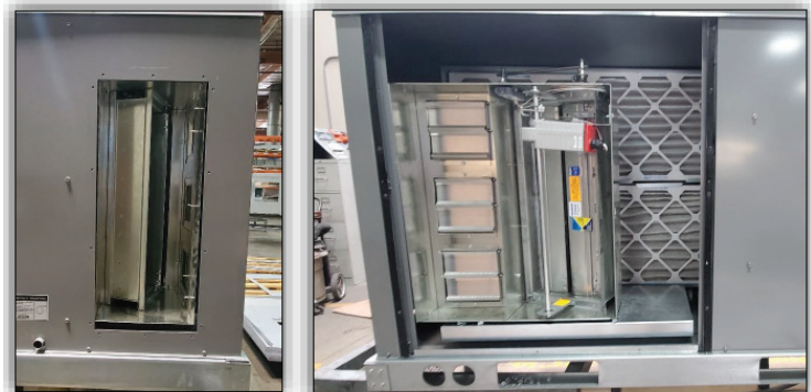
Figure 9: Insert the economizer (Step 4).
