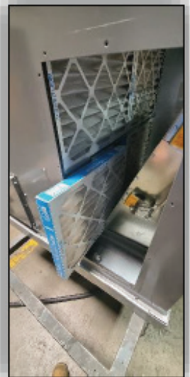
Figure 25: Pulling Out the Bottom Filter.
