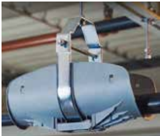
Examples of Piping Supports.
