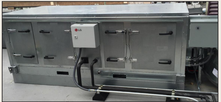
Figure 25 - Rooftop Air Handler
